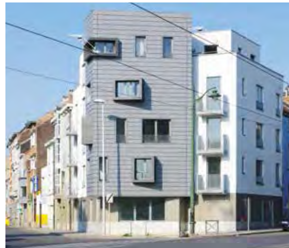
Appartementsblok in Brussel in handen van de Community Land Trust
